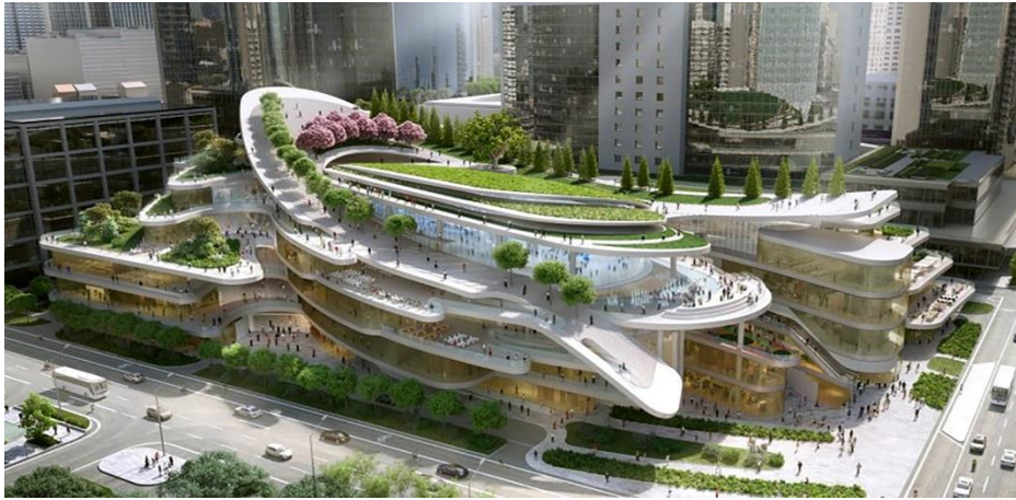
Figure 9. Roof garden in a Smart City (Based on Google Images 2019)
