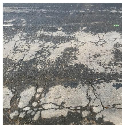
Fig. 8 Starting condition of a road in advanced degradation status.
