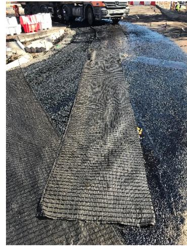
Fig. 12 Geogrid overlap poorly executed.
