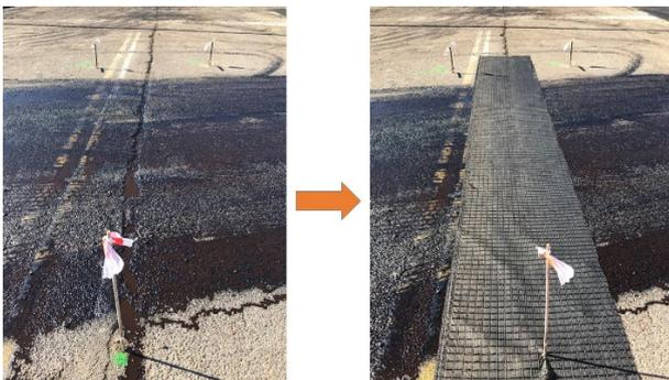
Fig. 11 Incorrect performance over a longitudinal cracking.
