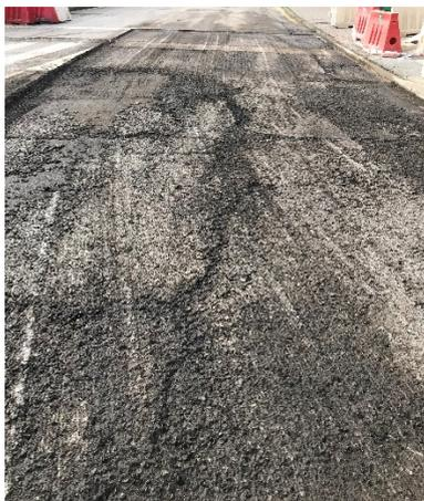
*Fig. 9 Deep cracks in milled pavement.*
