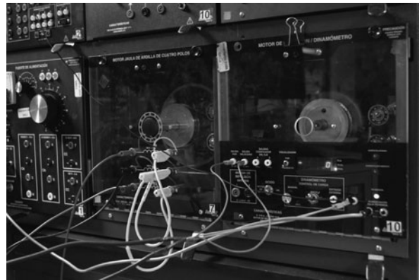
FIGURE 7. Induction motor-dynamometer group.
