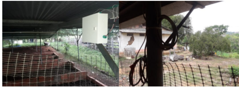
Figure 4. Installation and protection of the system control box.
