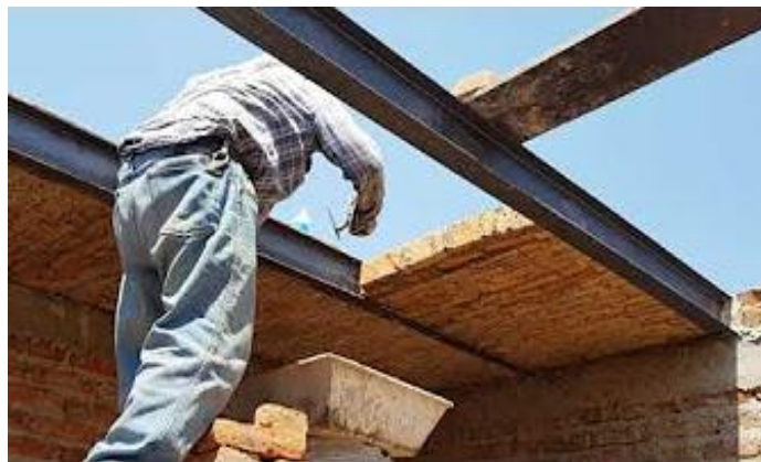
Figure 1. Vault ceiling construction
