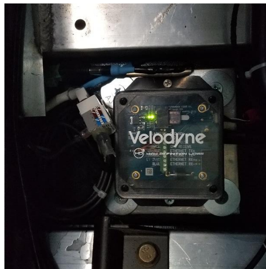
Figure 16. Front Velodyne Lidar VLP-16 box installed.
